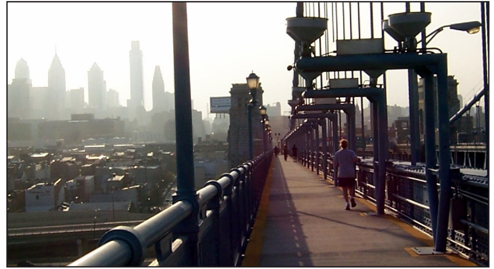
The Benjamin Fraklin Bridge Walkway
