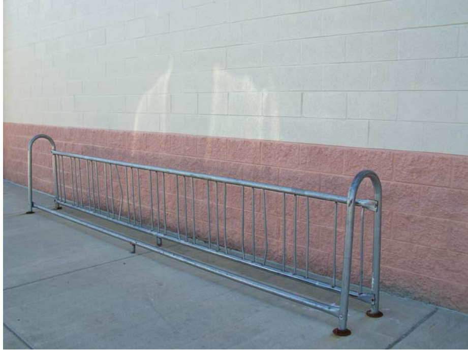
15. A frequent problem with school racks is that they are placed too close to a wall, preventing the bicycle from being put through the racks. (Photo of Acme at 19 th and Oregon by Jill Minick)
